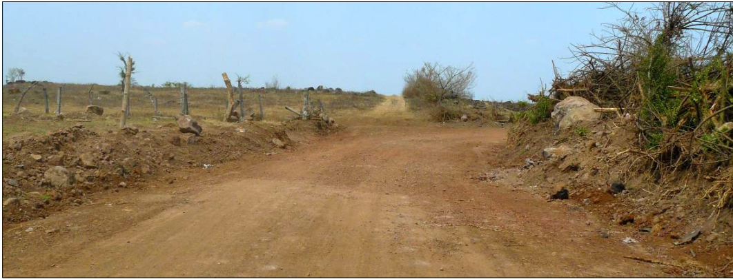
The new access road. This road and its branches extend for over 1,300 meters (0.8 miles), with a width of 10 meters (33 feet). The bulldozers graded down to the culturally sterile reddish subsoil, destroying archaeological deposits including structures, along its route.
