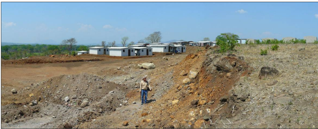
The housing project. In this area the bulldozers cut to depths greater than 3 meters (10 feet).
